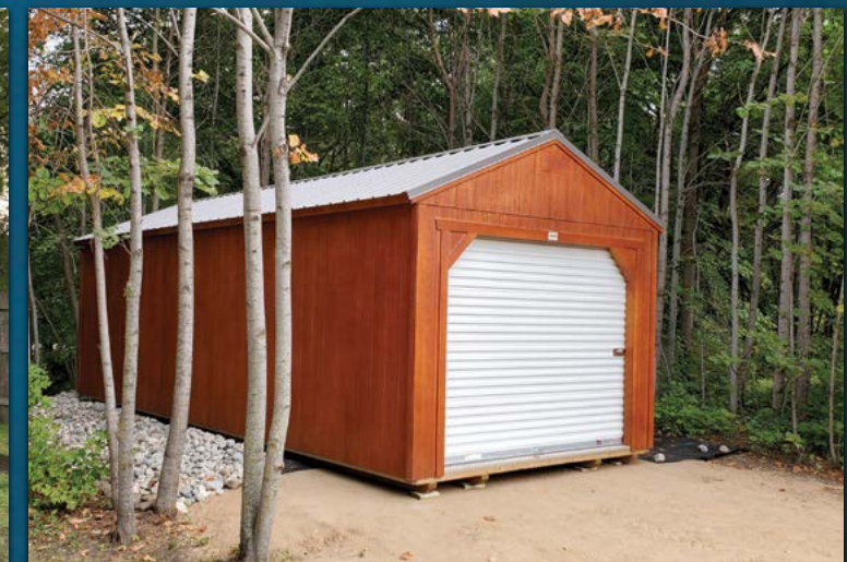
UTILITY GARAGE PACKAGE / PEWTER GRAY METAL ROOF MAHOGANY URETHANE ON LP SMART PANEL SIDING
